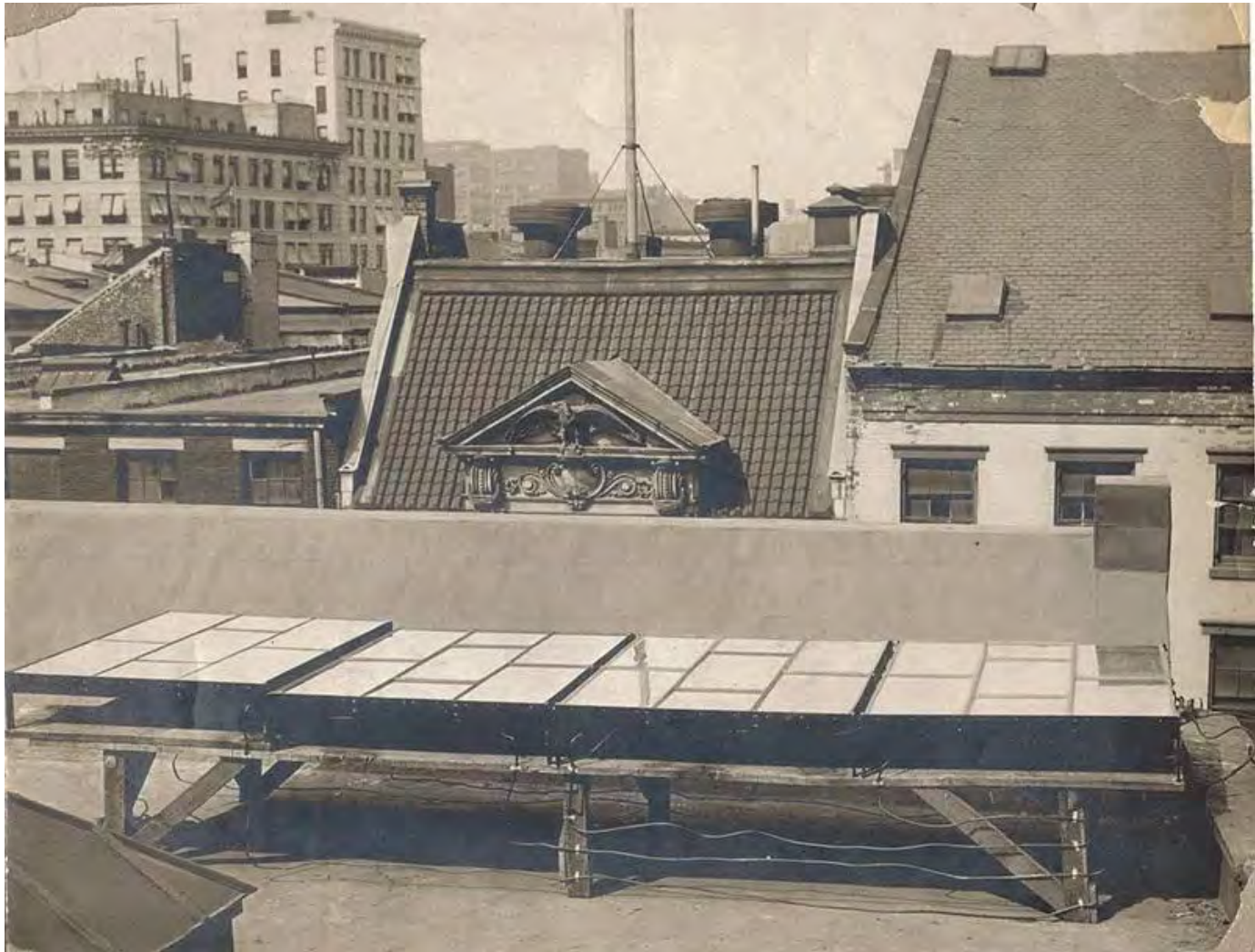
Charles Fritts installed the first solar panels on New York City rooftop in 1884. Courtesy of John Perlin
